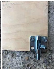
13. Place the 1.5" x .5" shim underneath receiving end of the barrel bolt and screw both into place.
